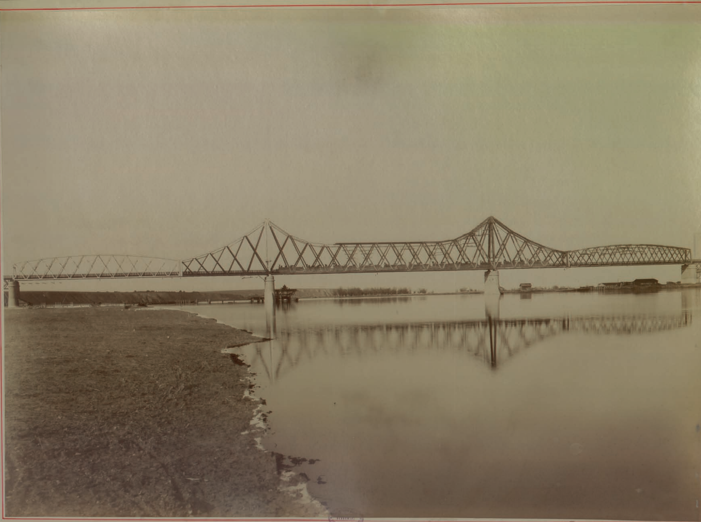
View of the bridge from the river bank
